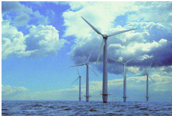
Fig. 6. An offshore wind farm
