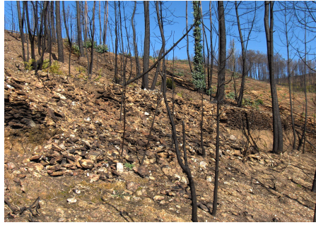
Photo 5. Destruction of terrace retaining walls due to fire and abandon of traditional agriculture in the “freguesia” of Ceira. (The photo was taken in February 2006)
