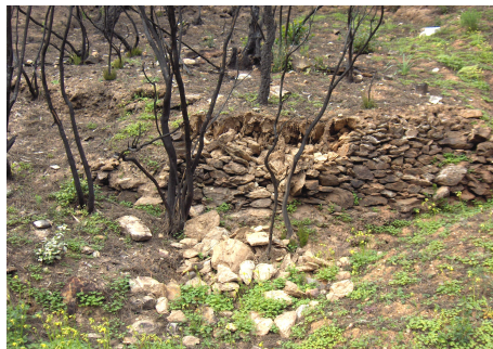
Photo 4. Destruction of terraces due to fire and abandon of traditional agriculture in the “freguesia” of Ceira. (The photo was taken in February 2006)
