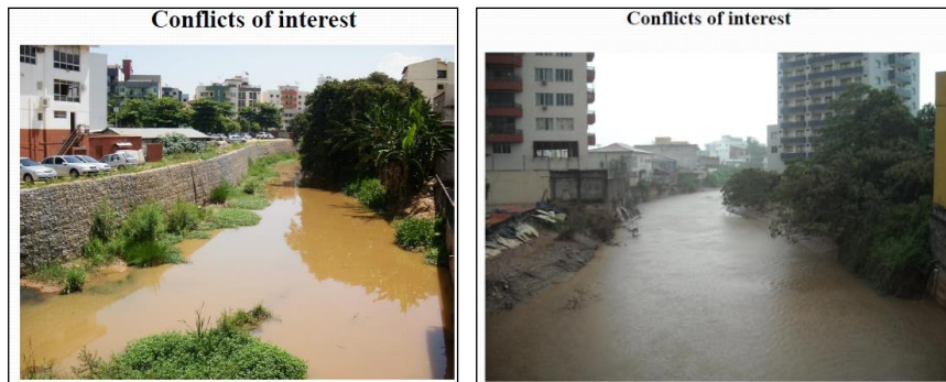
Figures 8 , 4 - Building too close to the river bank.
